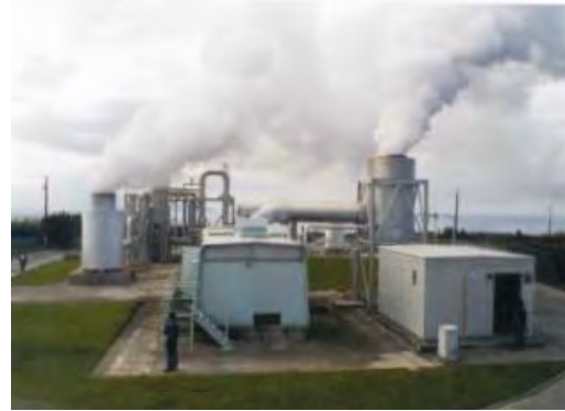
Fig. 8.48 Direct-intake, non-condensing single flash geothermal power plant at Pico Vermelho (São Miguel Island, Azores) exhausting steam to the atmosphere. (source: [2004Lun b ]).
