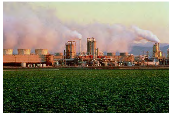
Fig. 8.51 Wet steam geothermal power plants with triple and dual flash cycles (left to right): Wairakei, New Zealand (with prawn pond in foreground) and Imperial Valley, USA, respectively (source: [2001Ano d ; 2002Ano]).
